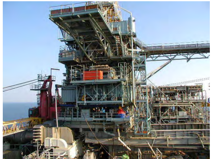
Figure 7 – Ram Powell rig after moving 60 feet to the west from storm motion
