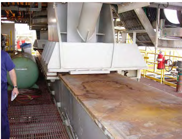
Figure 7 - Holstein Skid Beam
