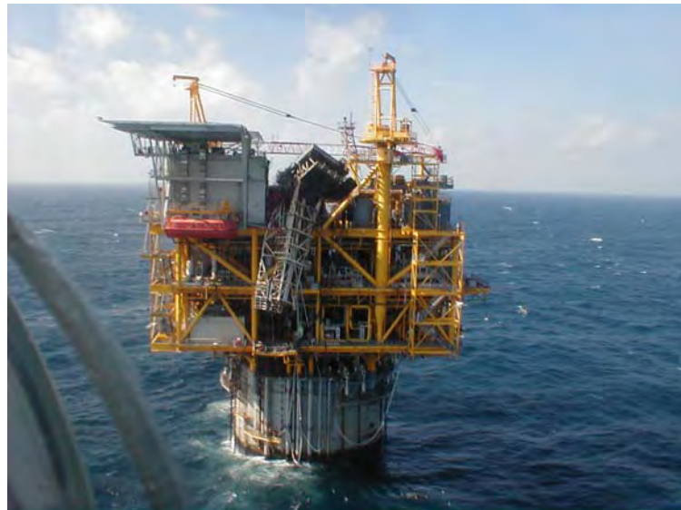
Figure 1 - Side View of Medusa Platform after Hurricane Ivan
