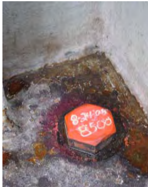
Figure 3 – Bolt After Torque Is Complete
