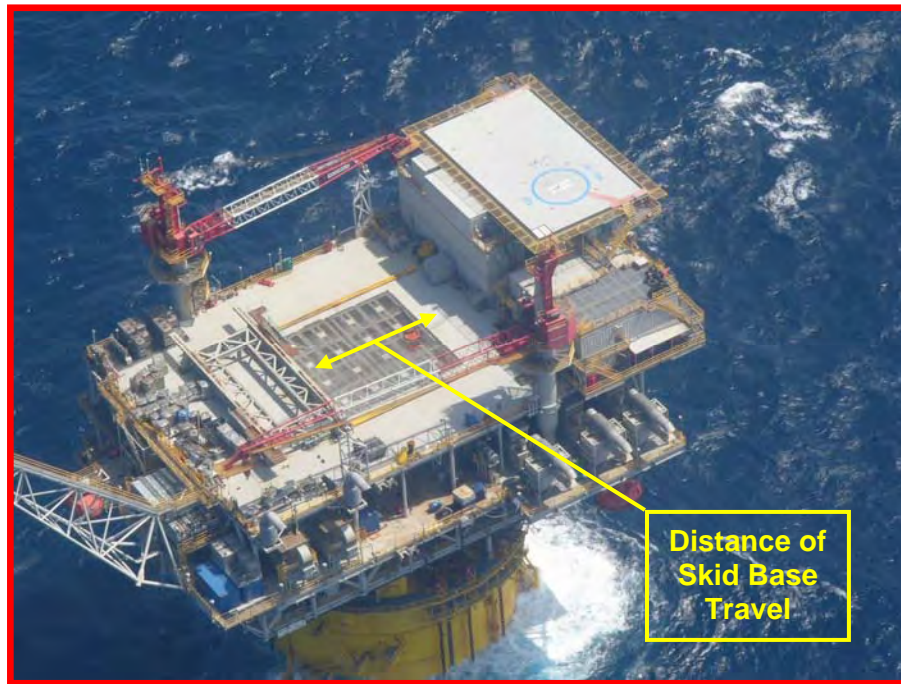
Figure 15 - Horn Mountain Aerial View Showing Rig Skid Base Off Skid Beams
