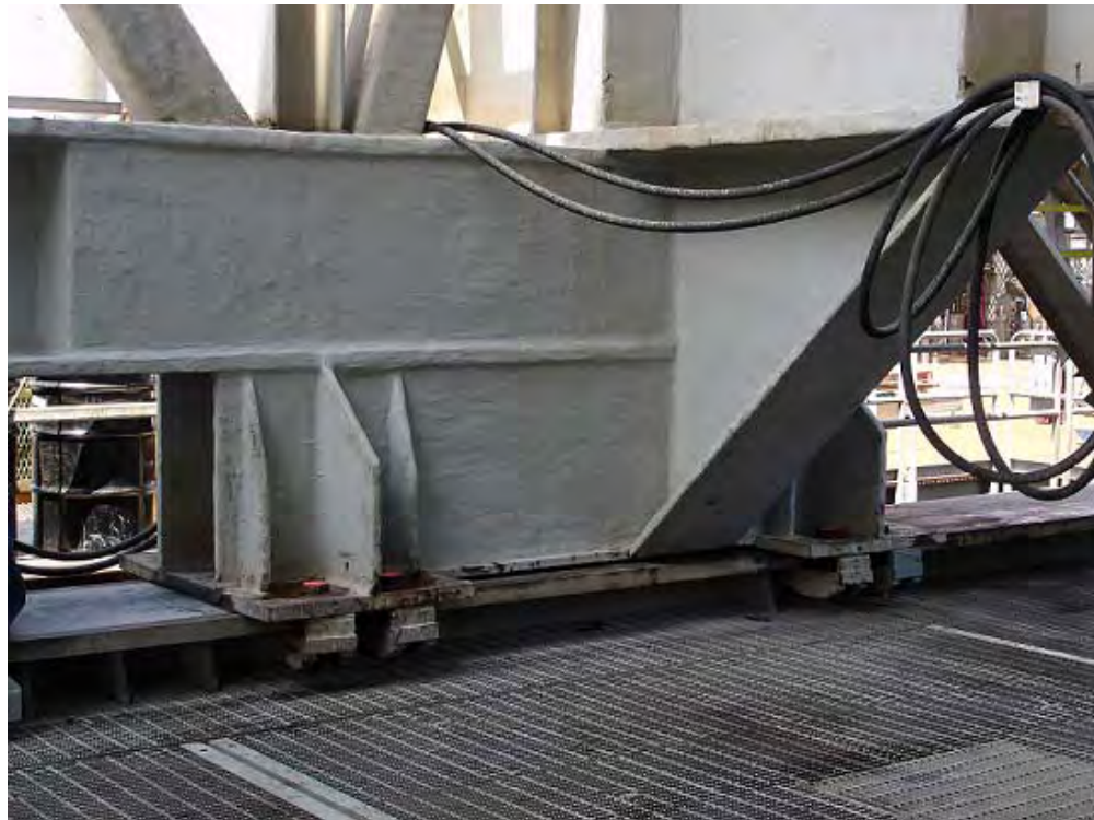
Figure 6 – Corner of Rig Substructure on Skid Beam
