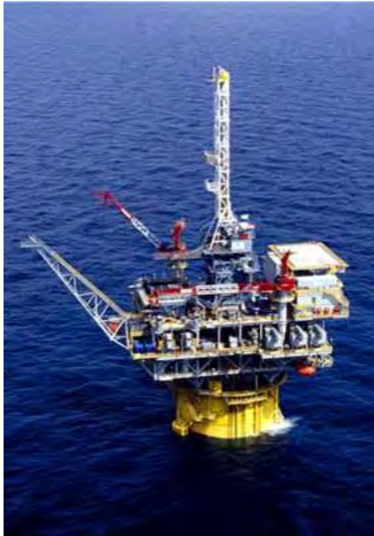
Figure 14 - BP Horn Mountain Platform with Drilling Rig on Board Prior to Hurricane Ivan
