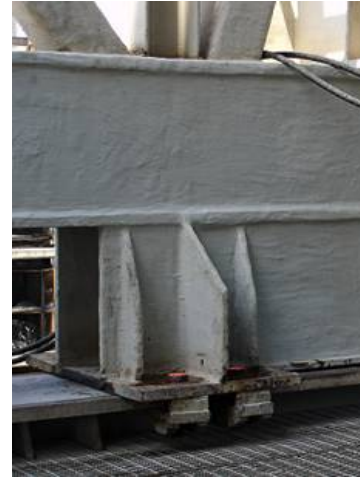
Skid Beam to Deck
