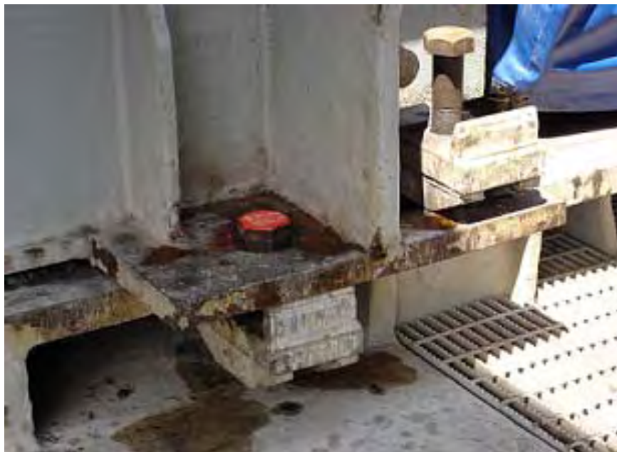
Figure 4 – Tie-Down Bolt on Clamp
