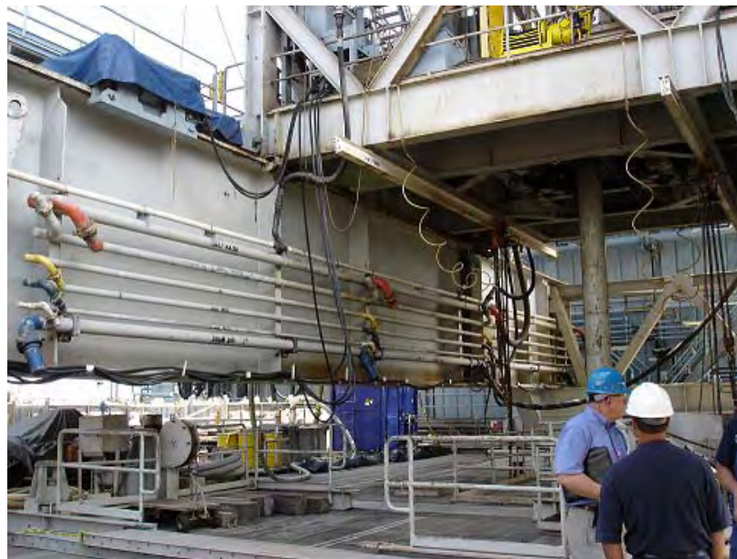
Figure 8 – Drill Floor on Substructure
