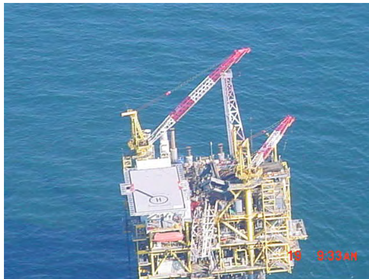
Figure 2 - Overhead View of Medusa Platform after Hurricane Ivan
