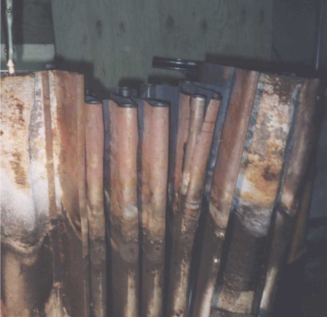
Figure 9-3. Crack in Pleat Material of Connector 1 after 500,000 Cycles with a 15-cm (6-in.) Stroke.
