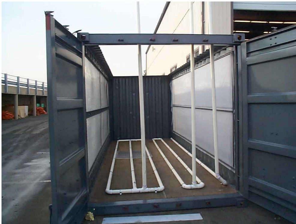
Figure 15: View inside container through open doors.
