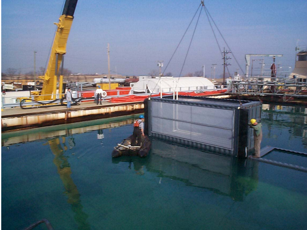
Figure 17: Containers being lifted into place across tank.
