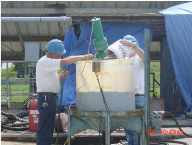
Figure 9: Mixing PAC into water in portable tank.
