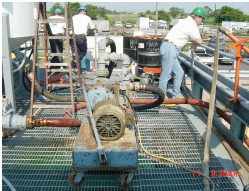
Figure 6-8. Main Bridge oil tank and Moyno distribution pump manifold
