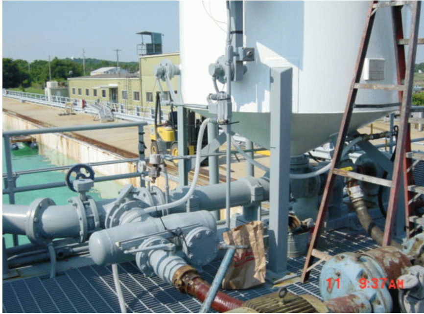
Figure 6-8. Main Bridge oil tank and Moyno distribution pump manifold
