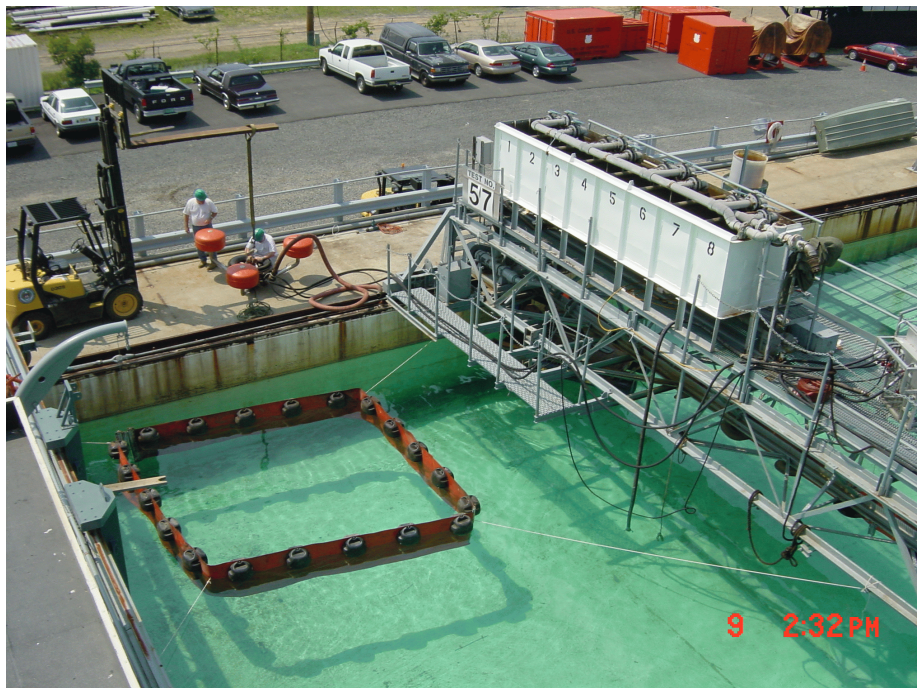
Figure 6-3. Recovery tanks on Auxiliary Bridge
