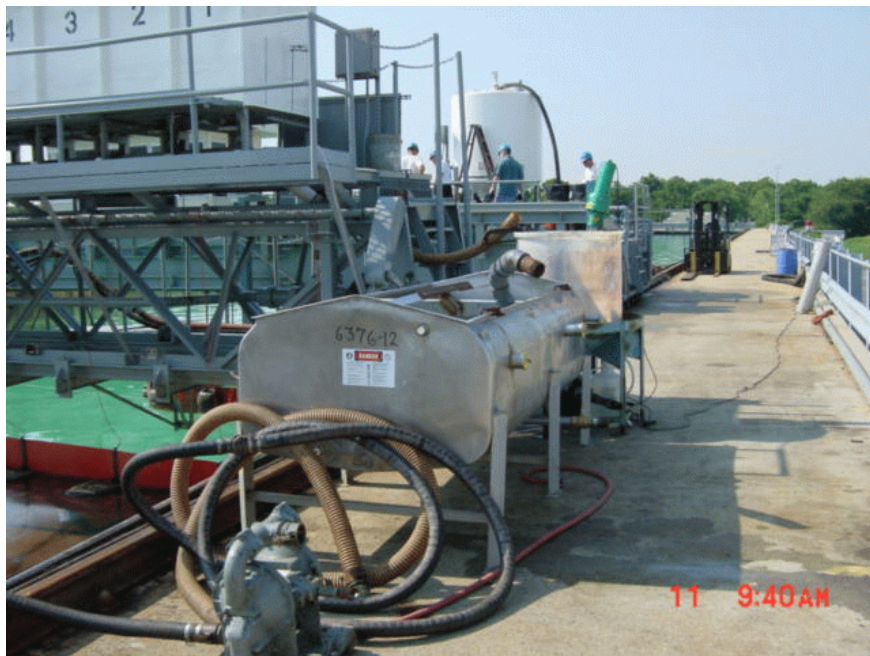
Figure 6-5. Steel temporary holding tank for decanted water.
