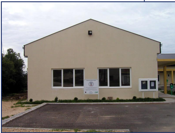
Vidrovan's new community center hosts a gym and plenty of public meeting space.
