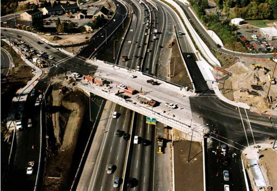
Figure 15: The Sylvan Road Bridge over U.S. 26 east of Portland utilized high-performance steel, one of the materials included in the IBRC funding program.
