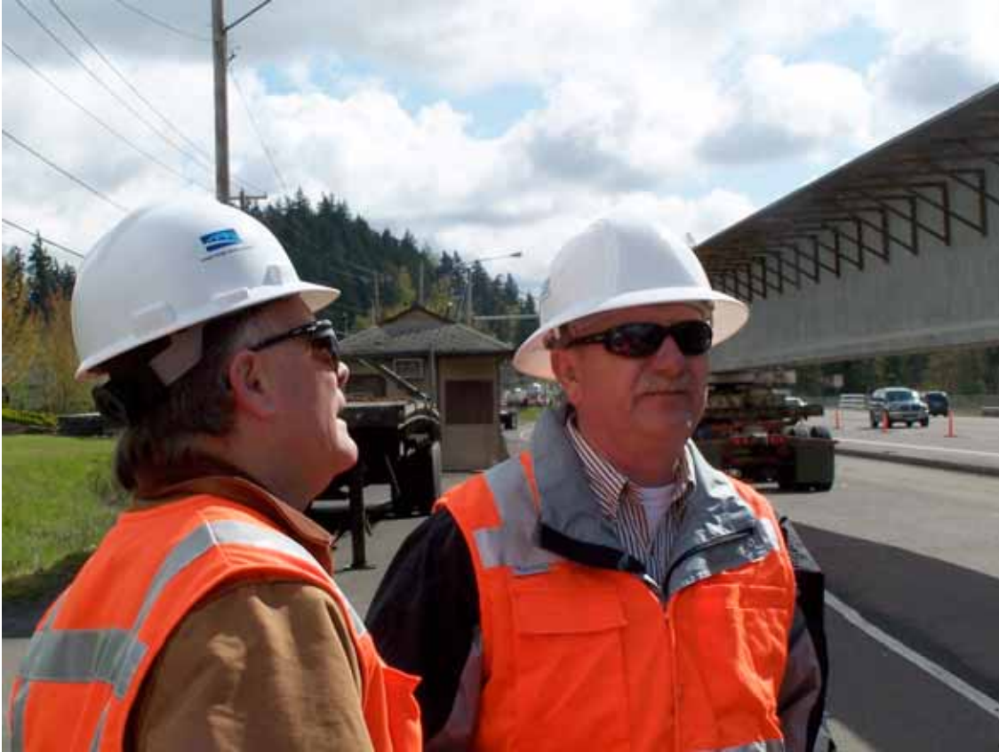
Figure 7: OTIA III State Bridge Delivery Program Health and Safety Manager Randy Peck and Quality Manager Jim Tew look over one of the Rock Creek Bridge beams being set as part of the Mt. Hood to Chemult project.
