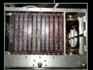
Multiplexer/Demultiplexer Mass Memory Unit (MMU) Processor Data Cards in U.S. Lab
