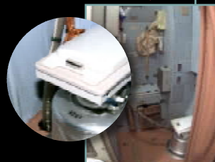
Toilet in Waste Management Compartment
