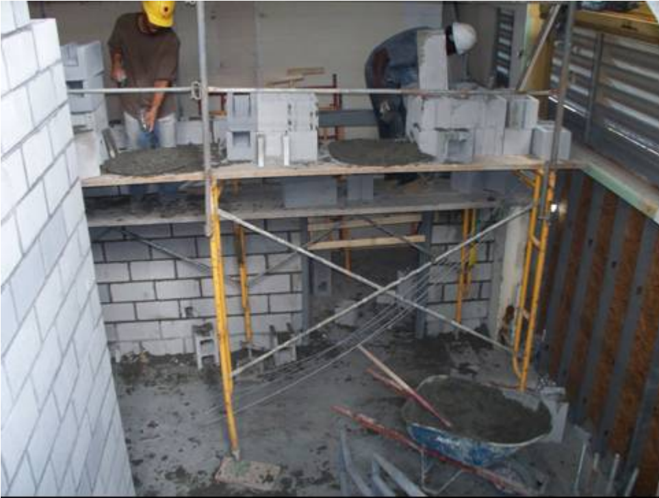
Block work Phase II. Downstairs Corridor
