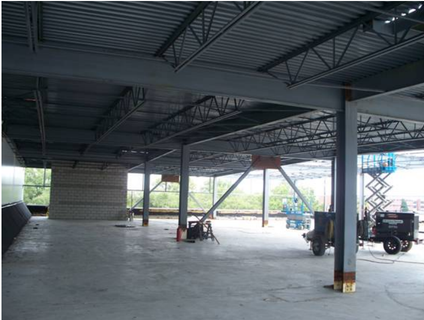
Steel Work and Block Wall Phase II.
