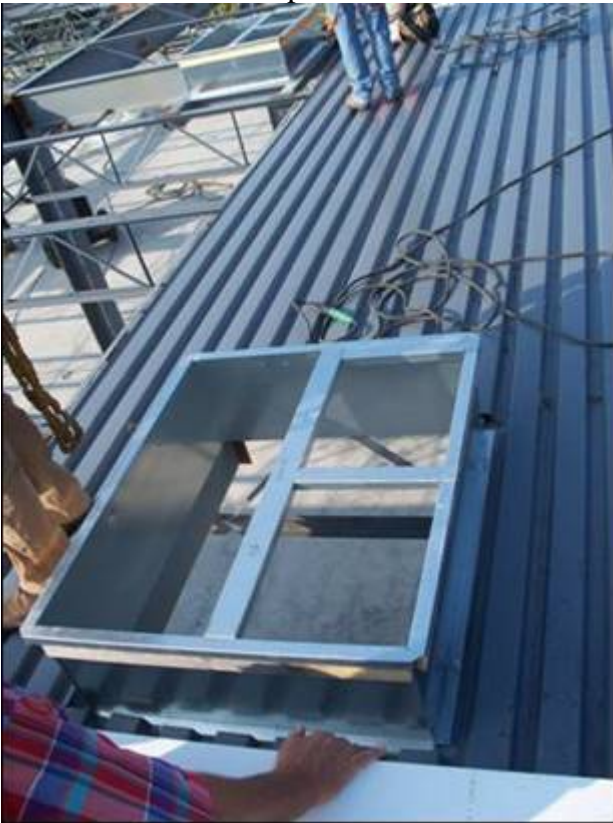
Roof HVAC Steel Preparation.
