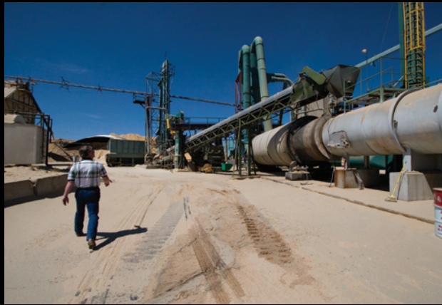
Dryer is fueled with scraps and defective pellets
