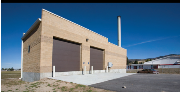
Wood-chip boiler building that heats the Darby School, the first Fuels for Schools project in Montana.
