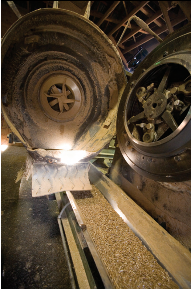
Pellet mill open for cleaning
