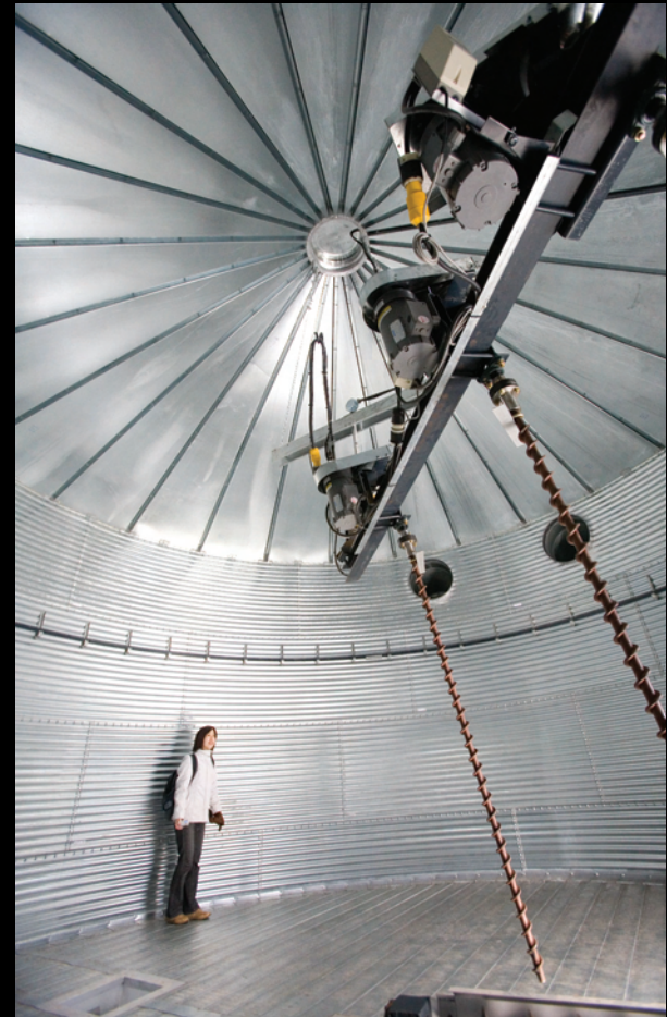
Grain silo ready for first batch of wood pellets
