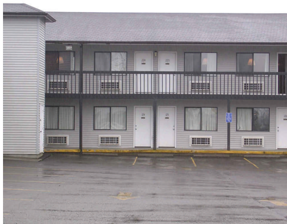
Western Royal Inn before motel was elevated to prevent repetitive flood damage.
