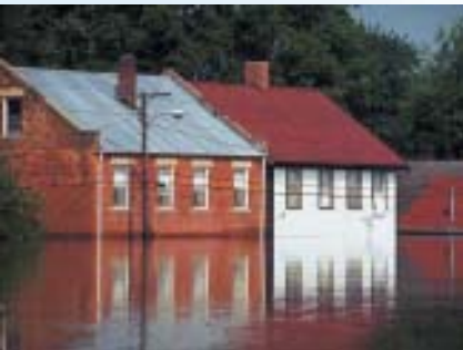
Floodwaters, Saint Genevieve, Missouri, 1993. (Photo credit: FEMA.)
