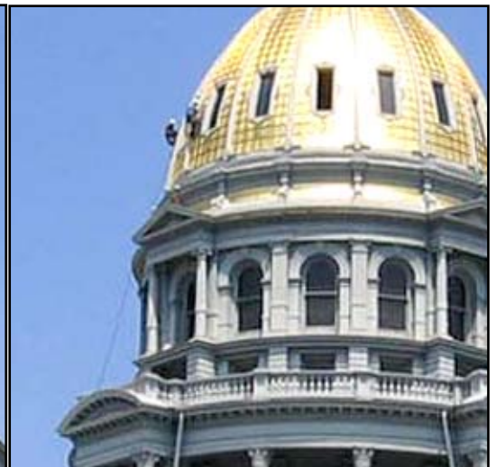
Workers recently conducted a "dome assessment" by rappelling down the sides of our State Capitol's dome. The assessment will provide information as to the overall condition of the outside of the dome, which hasn't had such a close inspection since the 1950s.
