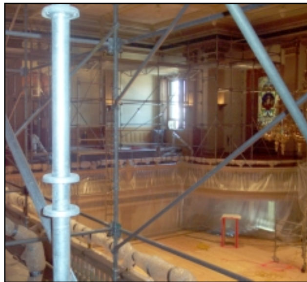
In the Senate Chambers great efforts have been made to protect the ornate woodwork and plaster that adorn the walls and ceiling.
