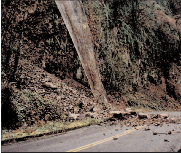
Landslides are a common problem in many areas of Oregon; they affect roads, houses, and the economic livelihood of communities.
