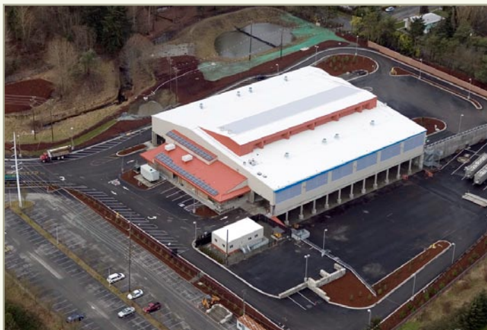
Shoreline Recycling and Transfer Station is the first of a new generation of transfer facilities.
