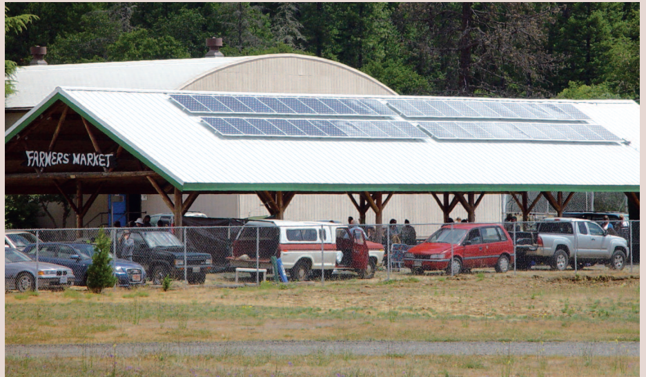
Selma Farmers Market vendors and patrons are sheltered under a solar-paneled roof. Photo Credit: Karen Chase.
