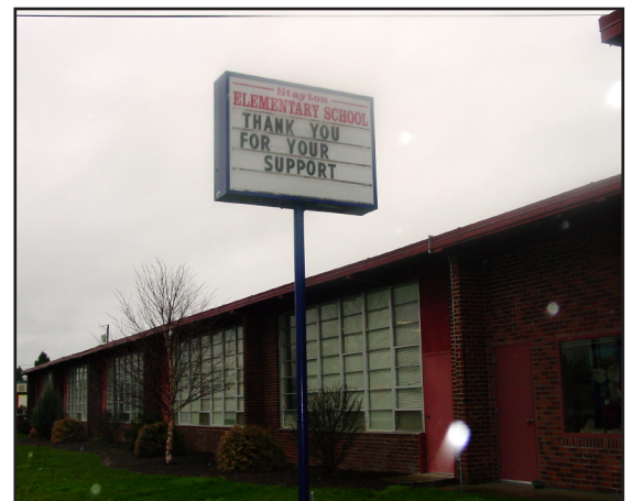
Stayton Elementary School and Stayton Middle School students, teachers and staff benefited from lighting and heating/cooling system improvements.
