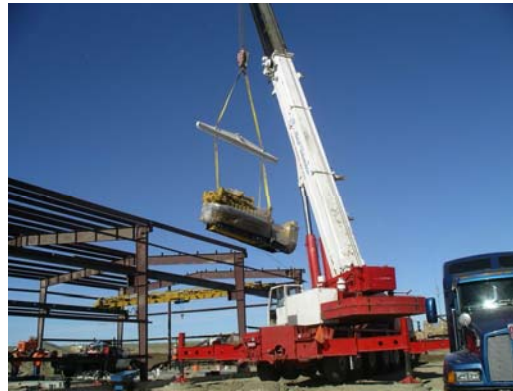
(Crane drops in a Caterpillar 3520 C generator on the Finley site.)
