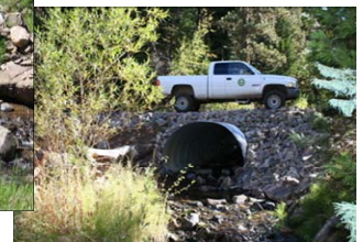
“Holgate Logging redesigned and installed culvert.”
