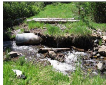
“Holgate Logging redesigned and installed culvert.”
