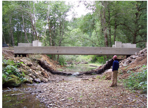
Concrete bridge installed over West Fork Millicoma
