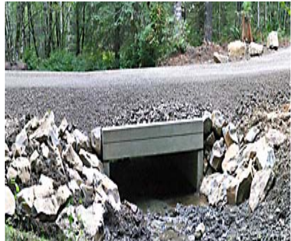
Sterling Ranch Road, open bottom, slab culvert
