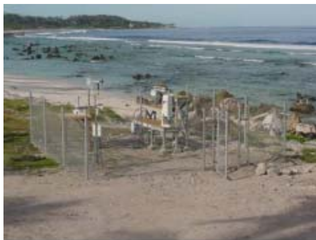
Figure 3. Existing facility at Nauru.
