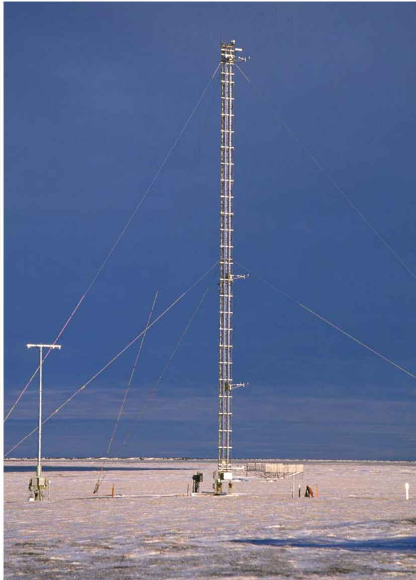
Figure 3. Met system tower at the NSA site in Barrow, Alaska.
