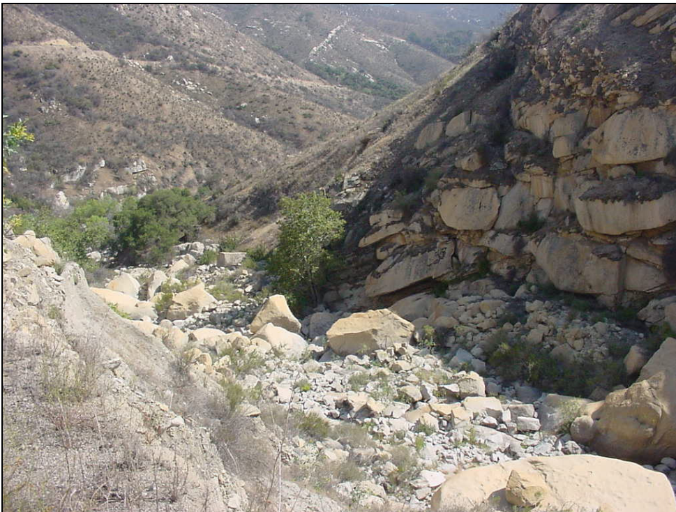
Figure 20. Photographs demonstrating loss of sediments below Loveland Dam.
