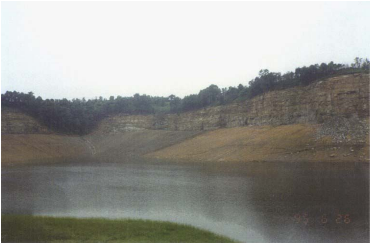
Photo 14. Seepage Barrier by 2000 Breakthrough (After Construction) - June 26, 1995. Source: GAI. The 2000 breakthrough area is located at the left-center of the photo. Pool elevation 1,006 feet msl. Mine roof elevation 973 feet msl. Contour bench elevation 1,075 feet msl.
