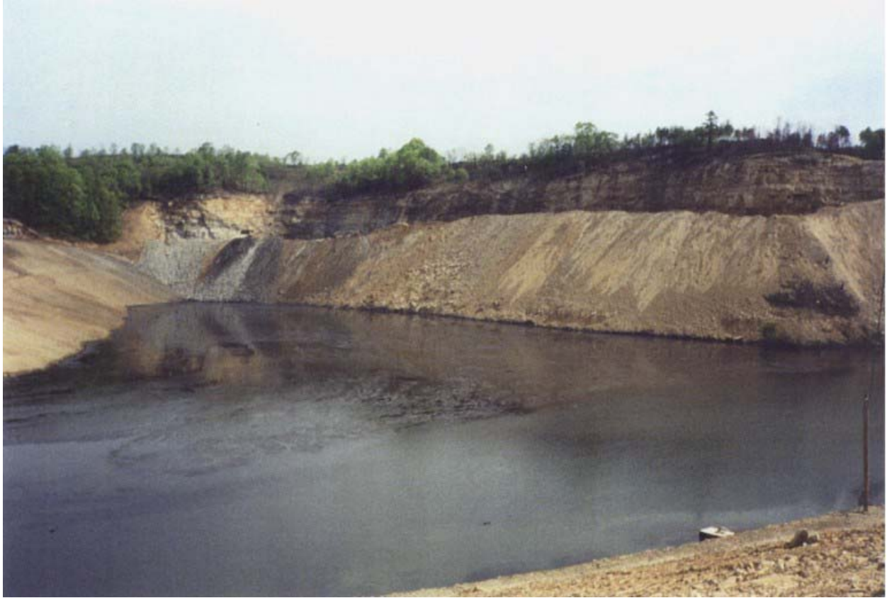
Photo 13. Seepage Barrier by 2000 Breakthrough (During Construction) - June 8, 1995. Source: GAI. The 2000 breakthrough area is located at the left-center of the photo. Pool elevation 1,001 feet msl. Mine roof elevation 973 feet msl.
