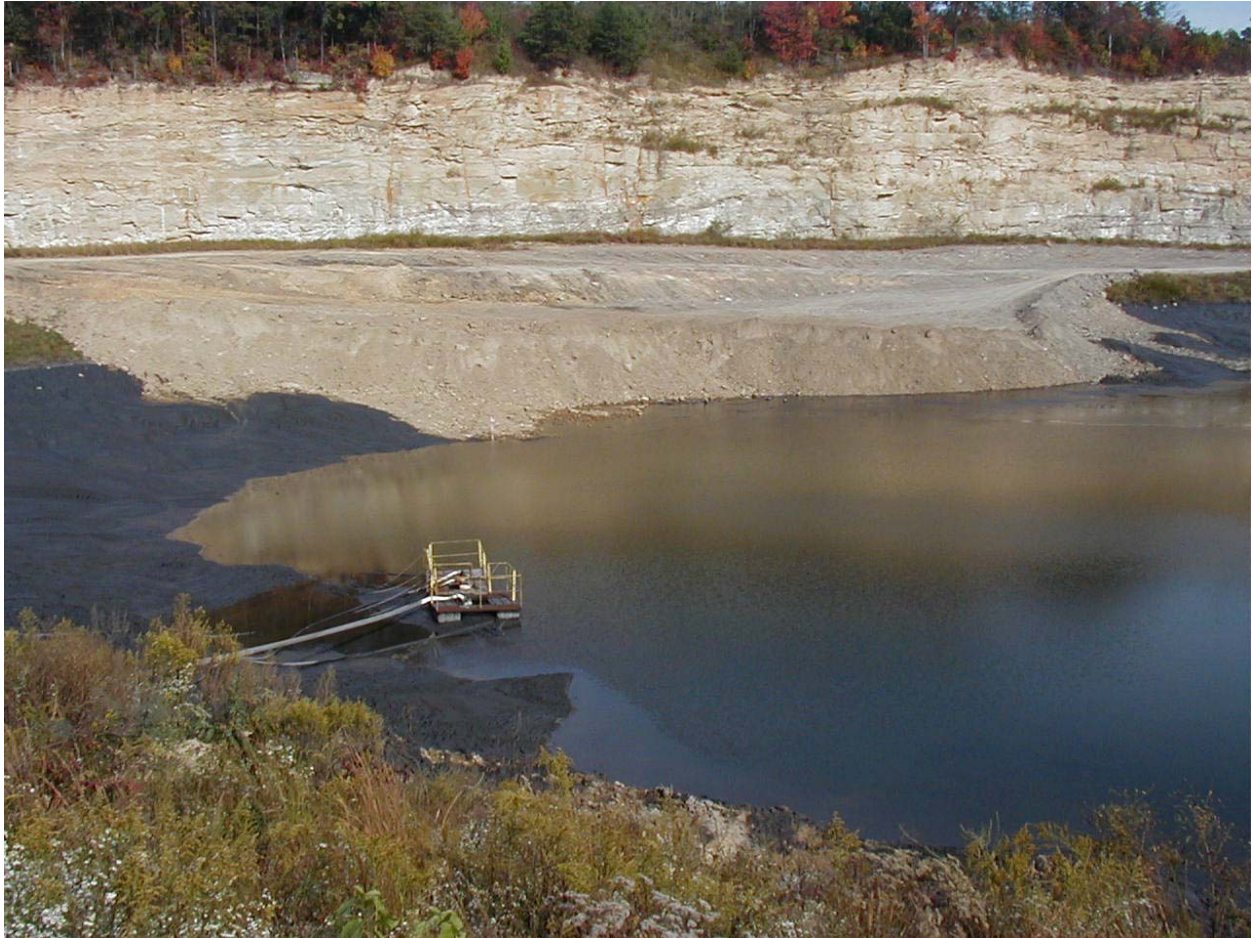
Photo 2. 2000 Breakthrough Area - October 16, 2000. Source: OSM. Pool elevation about 1,060 feet msl prior to breakthrough and 1,046 feet msl after breakthrough. Mine roof elevation 973 feet msl.
