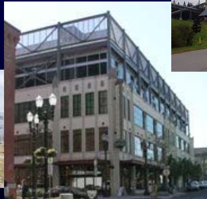
Portland District Cooling Co.
