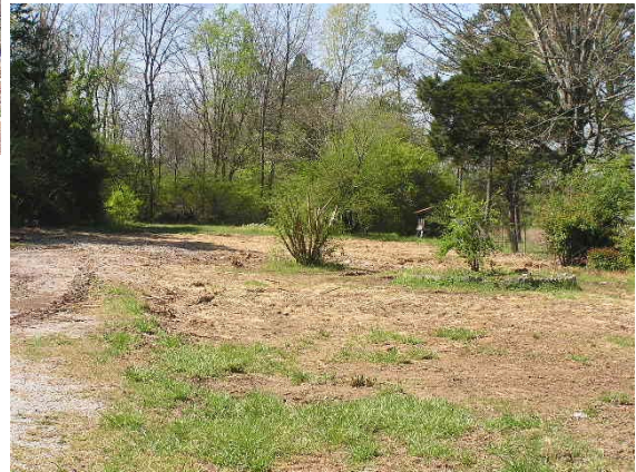
Below: 7456 Pinewood Drive, after demolition
