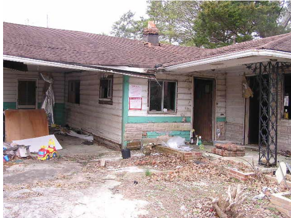
Above: 7456 Pinewood Drive, before demolition
