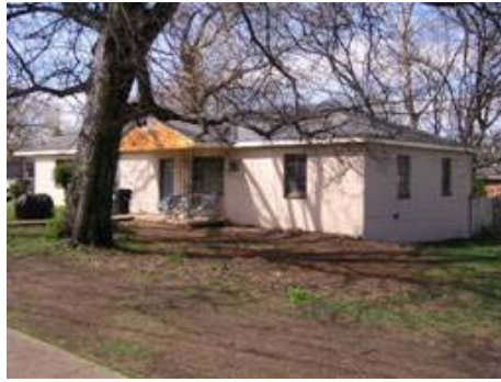
Above: 1823 Wilson Street, after
