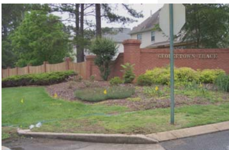
Before: Georgetown Trace Entrance
