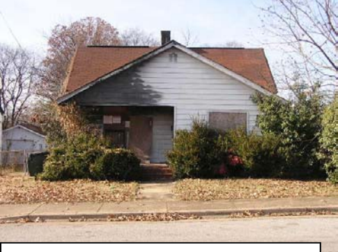
Before: 715 Arlington Avenue (exterior)
