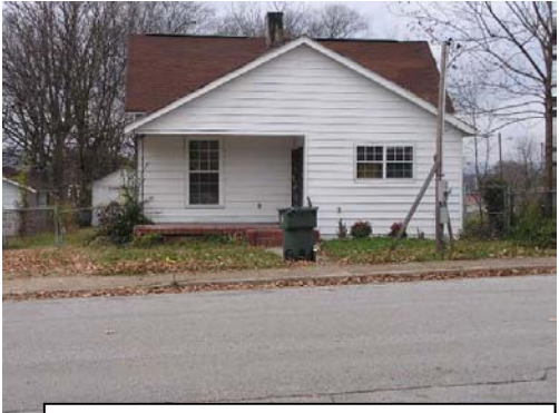
After: 715 Arlington Avenue (exterior)
