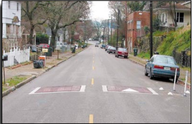
Speed cushions, such as these on Tremont Street, are one option available for neighborhood traffic management.
