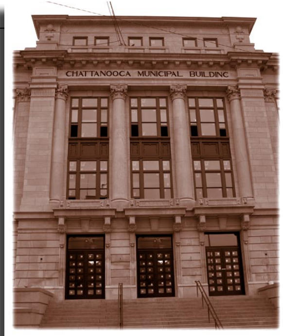
The Chattanooga Municipal Building, or City Hall, as it stands today.
