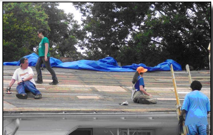
Student volunteers replacing a roof
