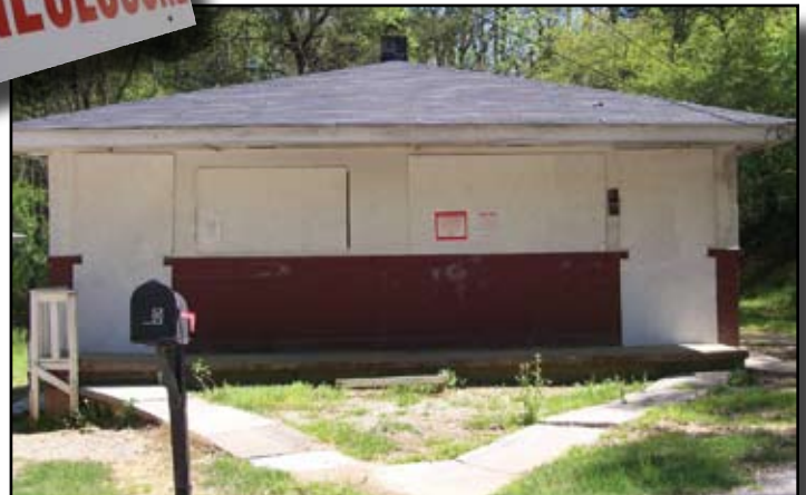
This duplex is a typical property that is in foreclosure.
