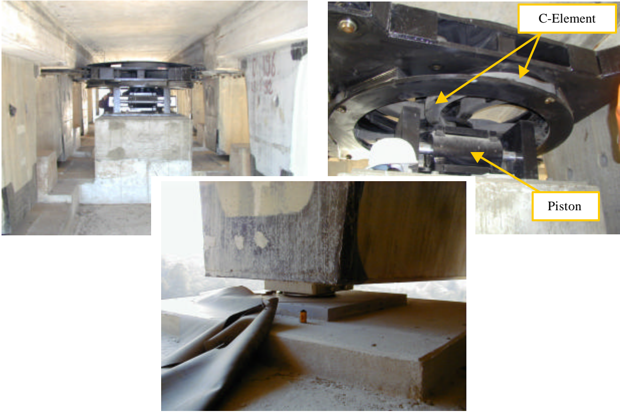
Figure 11. A pot bearing and an EDU unit.
