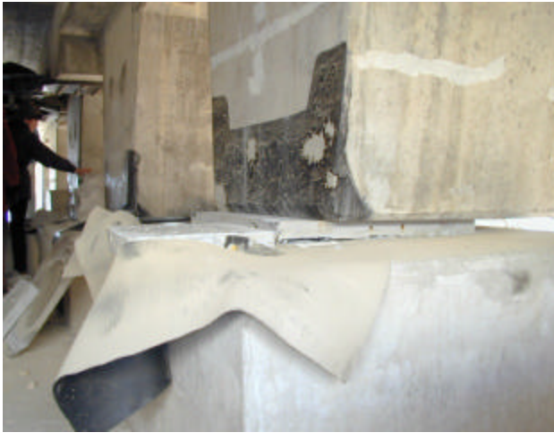
Figure 21. Bearing failure.
