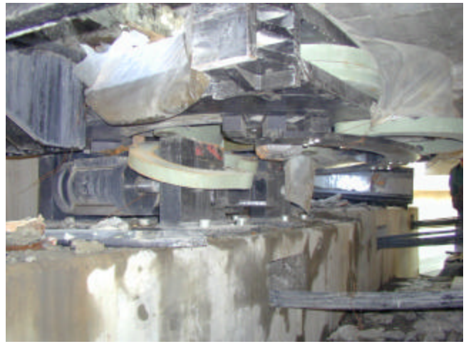
Figure 22. EDU failure.
