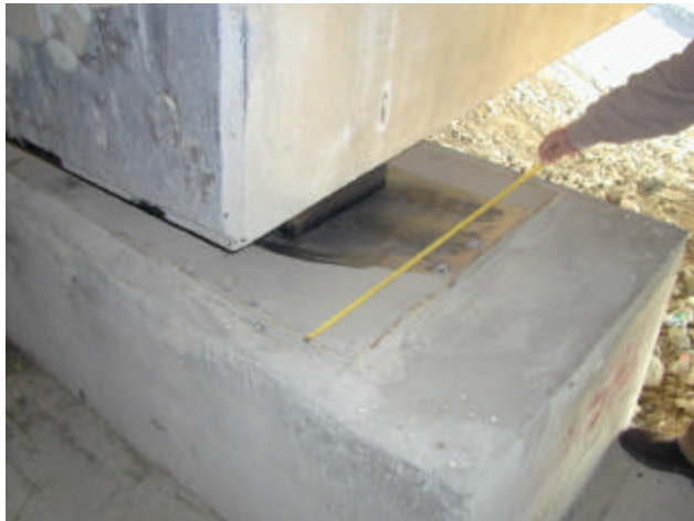
Figure 25. Well-proportioned, steel-reinforced elastomeric bearing pad showing evidence of translation.
