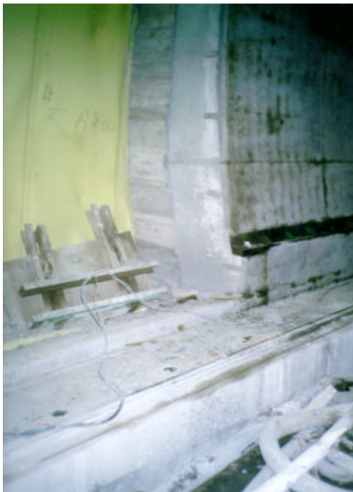
Figure 38. Completed concrete liner showing utility box beam.
