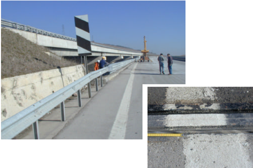
Figure 24. Translation of the eastbound span at the west abutment.
