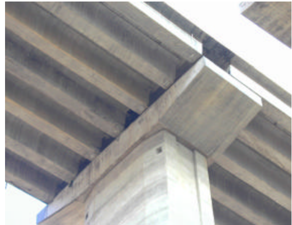
Figure 18. End of fascia girder extending beyond pier table.
