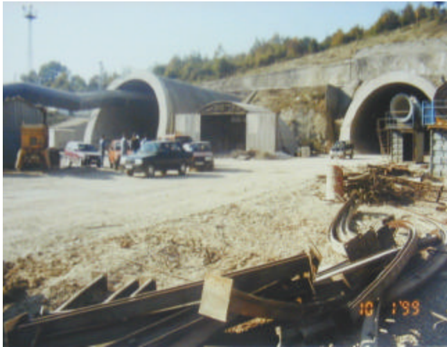
Figure 9. Bolu tunnel at the Elmalik portal.
