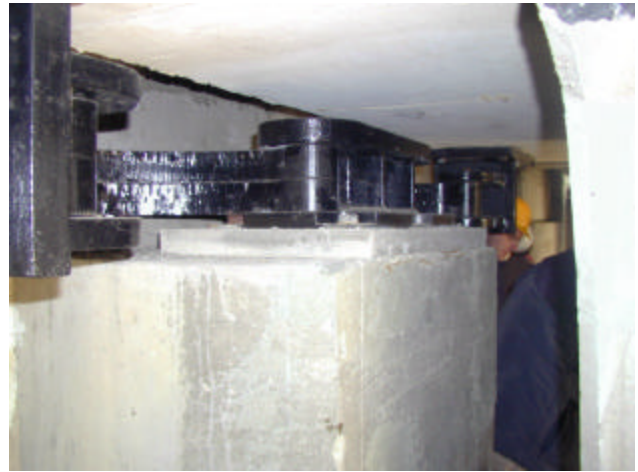
Figure 26. Flaked-off paint of an EDU C-element that had functioned properly.
