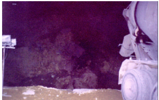
Figure 32. View looking at the collapse of the eastbound tunnel.
