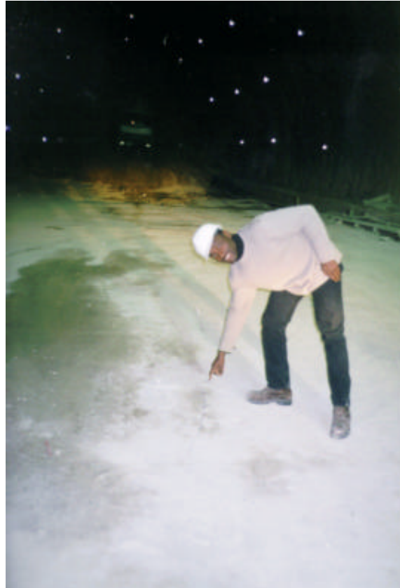
Figure 39. Longitudinal cracking above invert.
