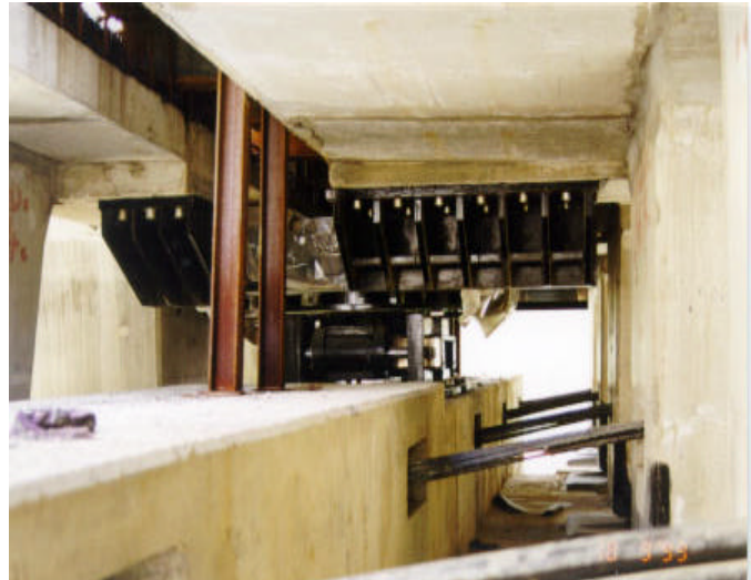
Figure 13. Cable restrainers at the expansion joint.
