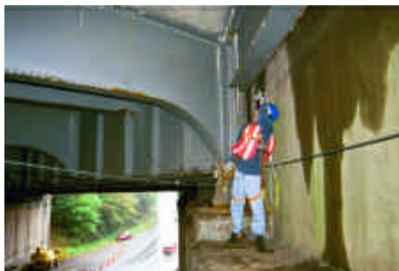
Inspector checking behind the end floor beam.
