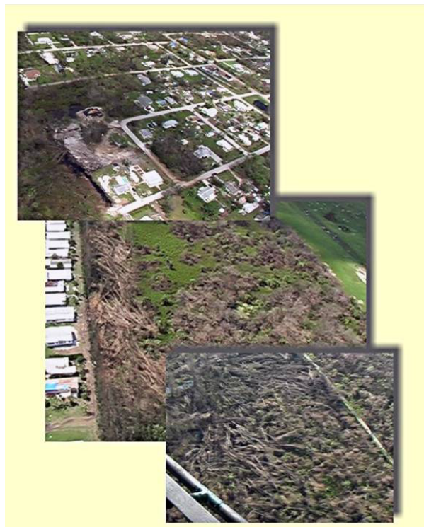
Fig. 9 Photographs of enhanced wind damage associated with Hurricane Jeanne taken from air surveys conducted by the authors. These tornado-like swaths of enhanced damage were observed in extreme Southern Brevard County and occurred as the eye-wall passed over the region. Tree and structural damage within the swaths was much greater than that observed immediately adjacent to the paths.
