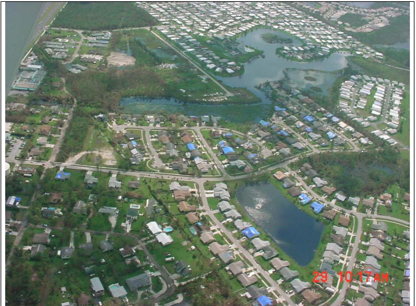
Figure 6 –Most common damage encountered, mainly scattered significant roof damage. (September 26, 2004 10:17 AM EDT)
