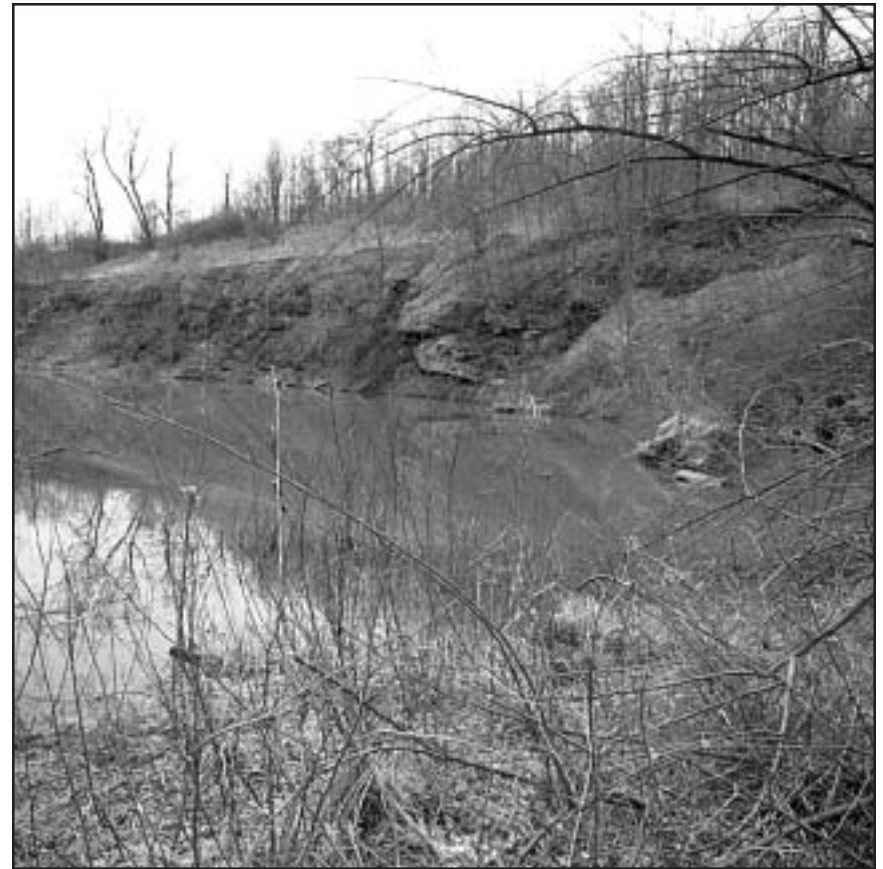
Abandoned surface mines may contain unstable highwalls -- where injury or death from falling rock creates serious danger. In addition, highwalls present a serious hazard to off-road vehicles, who's drivers may accidentally drive over the edge. The water-filled pits at this Midwest abandoned coal mine have steep, unstable banks and sharp rocks hidden under the water.
