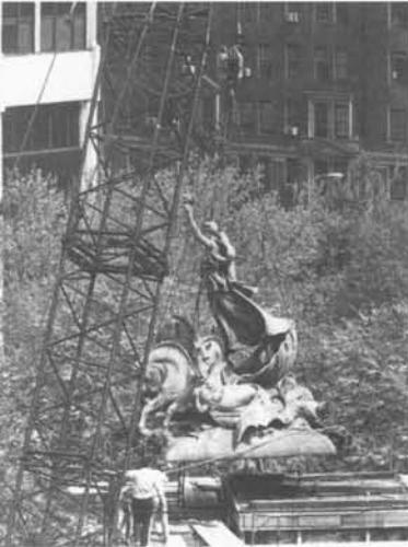
Members of Ironworkers, Local 197, Stone Derrickmen and Riggers hoist the 17-ton statue, Columbia Triumphant, to its base at Columbus Circle in Central Park, New York City, in 1980. Photograph from the Stone Derrickmen and Riggers, Ironworkers, Local 197, Collection, Robert E. Wagner Labor Archives.
