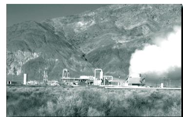
Geothermal energy is the natural heat of the earth. The Caithness Power Inc. geothermal plant in Dixie Valley, Nevada, converts extracted geothermal energy into electricity to meet a variety of human needs (photo by BLM).
