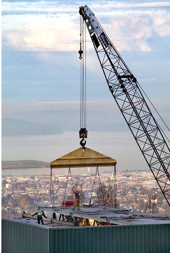
FIGURE 1.15 Demolition of facilities that are unsuitable for future research purposes
