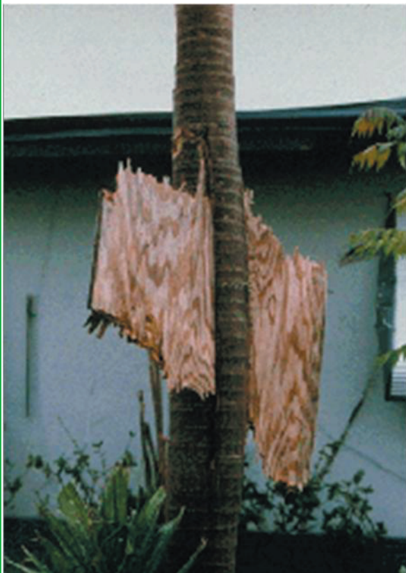
Hurricane Andrew wind damage in South Florida (August 1992)
