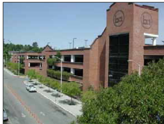
Figure 25: Walnut Creek Parking Structure
