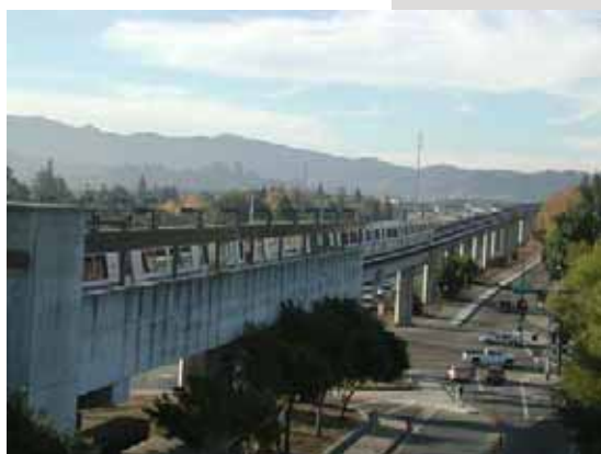
Figure 23: Walnut Creek Station Platform, looking north
