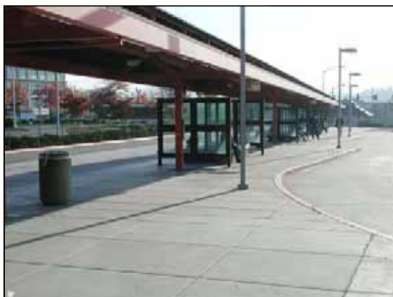
Figure 18: Walnut Creek Bus Intermodal Facility
