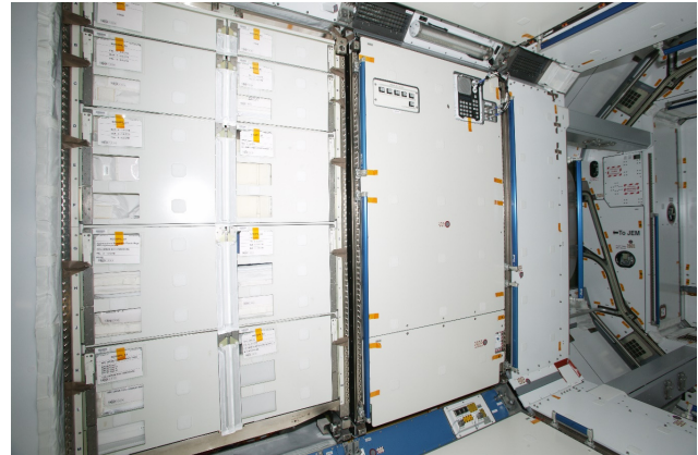
Node 2 will launch with 4 Avionics Racks, 2 Resupply Stowage Racks (RSRs) loaded with cargo, and 2 Zero-g Stowage Racks. Show here are the RSRs.
