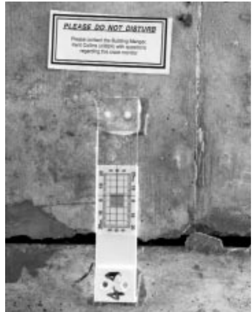
A crack monitor.
