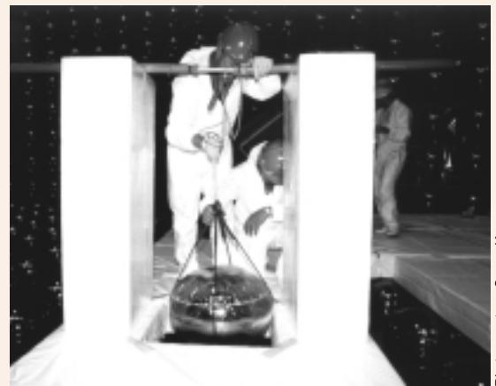
Workers installing a photomultiplier tube in the Super-K detector while it was down for maintenance. The styrofoam pads the workers are standing on are resting directly on top of other PMTs, and one of the theories on last year’s accident is that one of the PMTs was cracked during this process.
