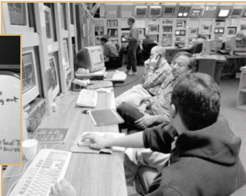
In the Main Control Room, operators have access to 90,000 read-outs and can control more than 40,000 devices related to the accelerators. Finding the optimal settings requires expertise and patience.
