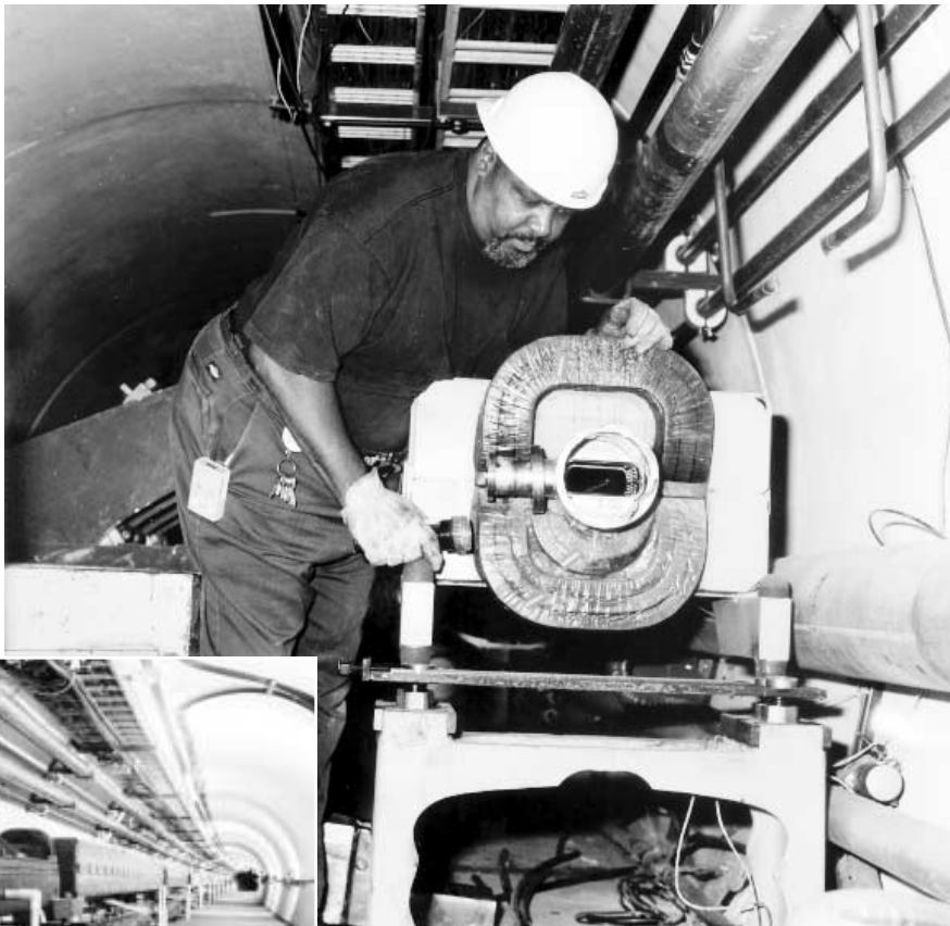
Theo Gordon, of the Mechanical Support Department, helps guide a magnet off its stand in the Main Ring and onto a flatbed lift.
